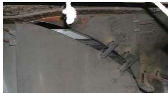
Figure 1. Actual crack of crane girder.
