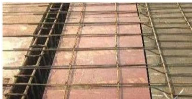
Fig. 3: Correct Spacing Of Slab Reinforcement
