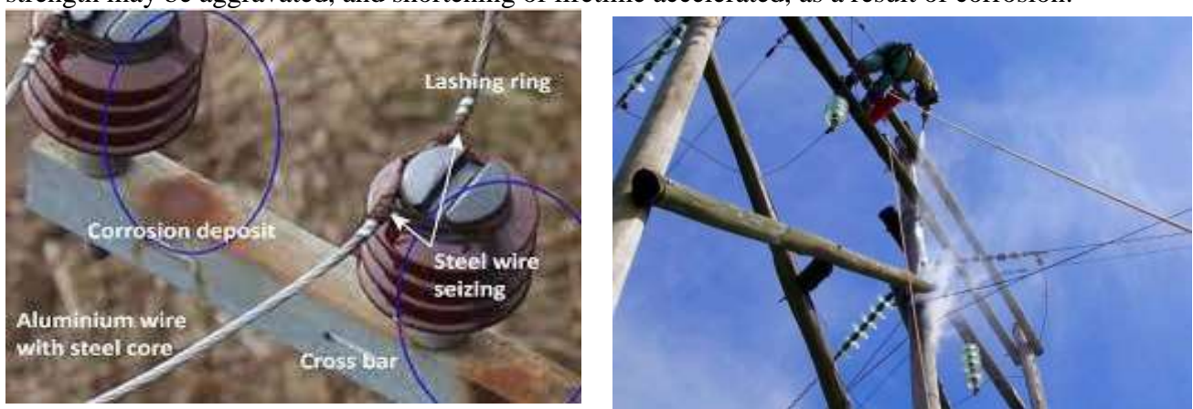
Fig :8.3 Fault insulator
