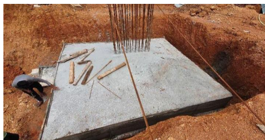
Figure 7: Completed RCC work
