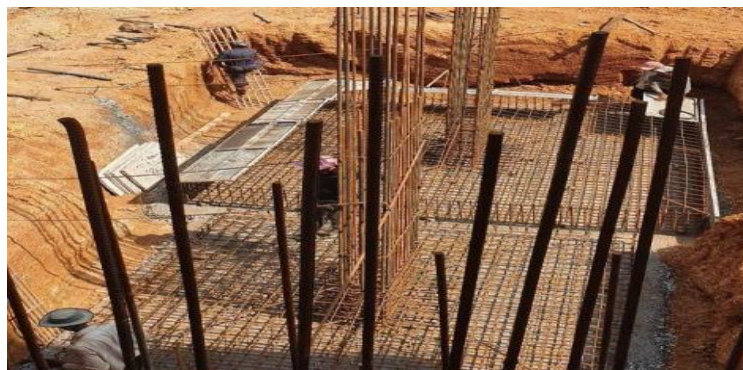
Figure 6: Laying reinforcement bars
