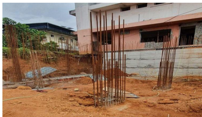
Figure 8: Completed Footing
