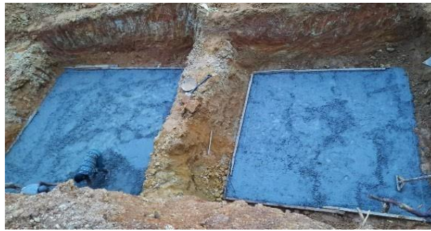
Figure 5: Placing PCC
